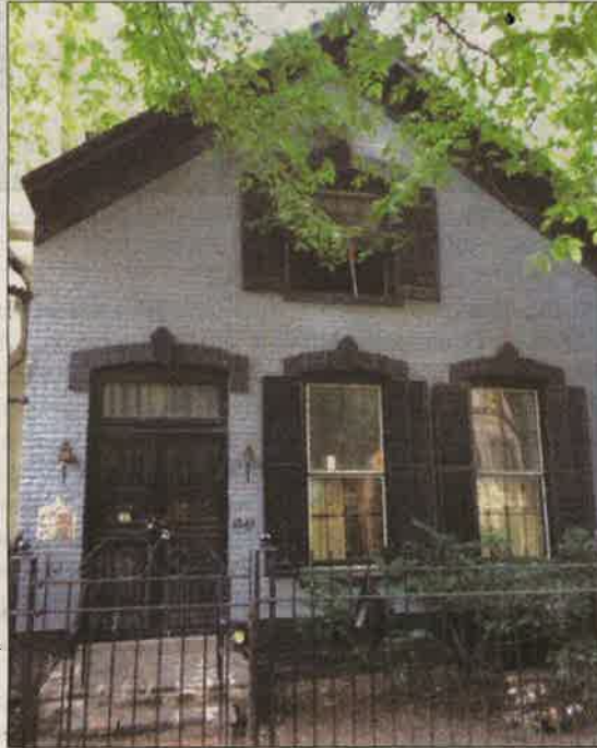
This orange rated building at 1241 N. State is in danger of the wrecking ball.
